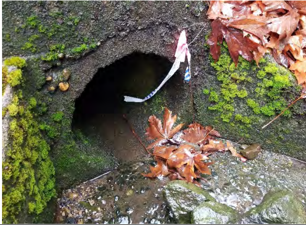
Culvert at N Mercer Way.
